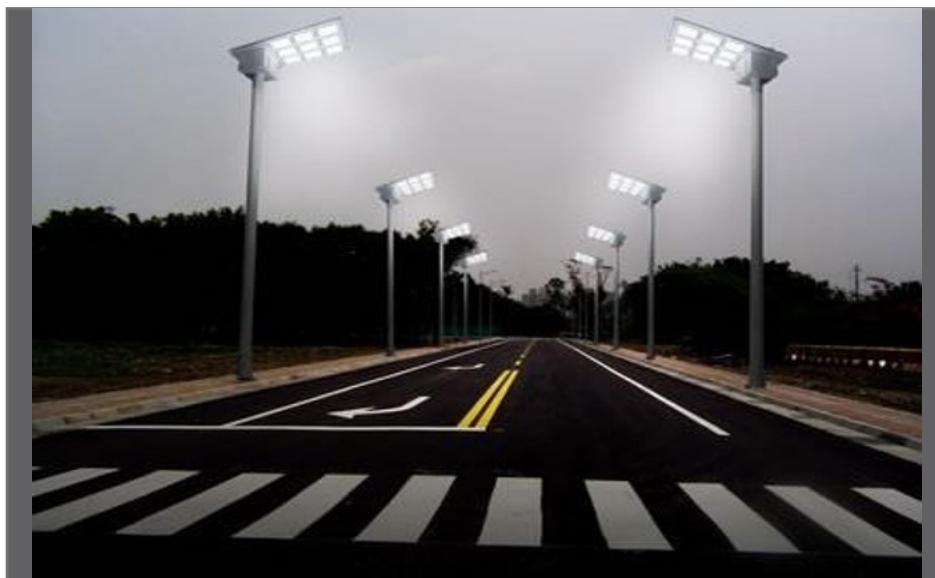
Fig. 1. LED street illumination
