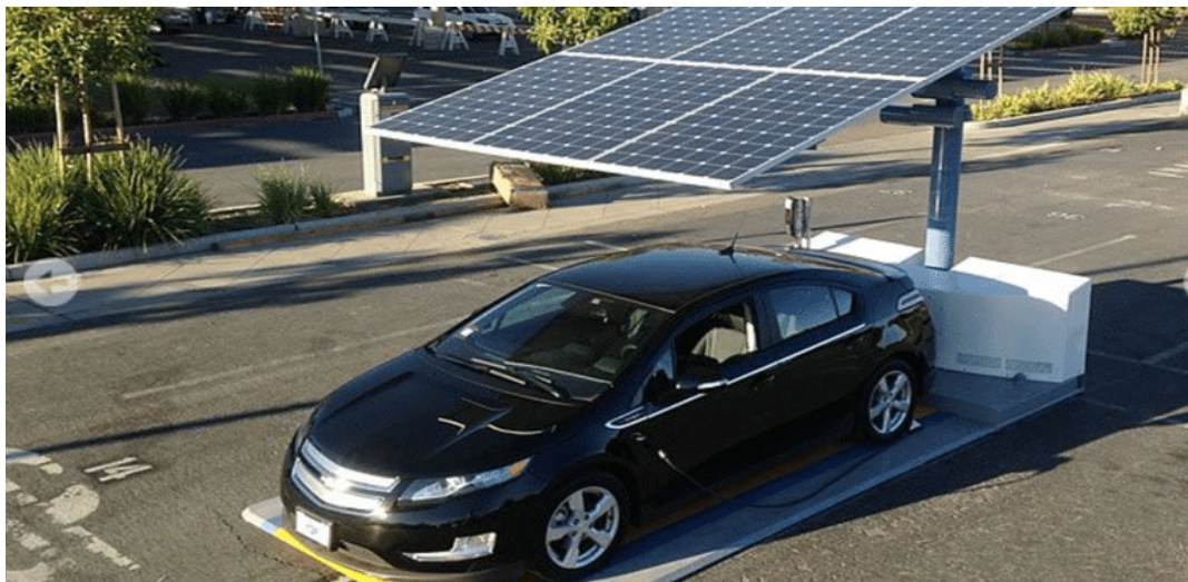
Fig.3. Solar Charging Station
